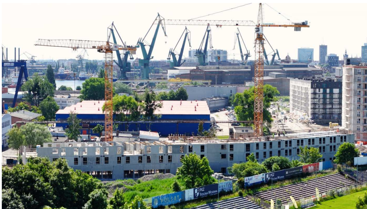
Student Depot, Gdańsk, budowa
